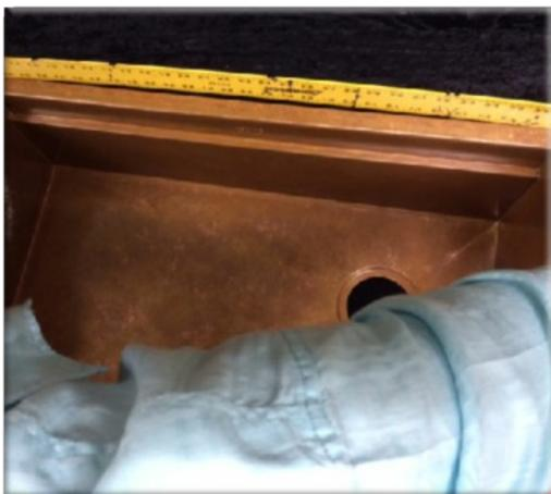
STEP ONE: Check the back of the sink to make sure it is straight. In this case, the back is bowed in. The fix is simple.
