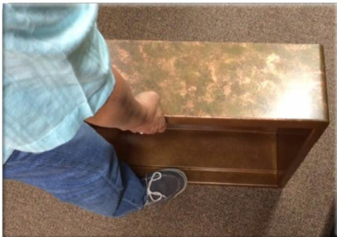
STEP TWO: Simply set the sink on its back. Place your foot in the center and pull up on the apron. You will likely have to pull quite hard. You will likely have to repeat this step. Don't worry, you will not damage the sink.
